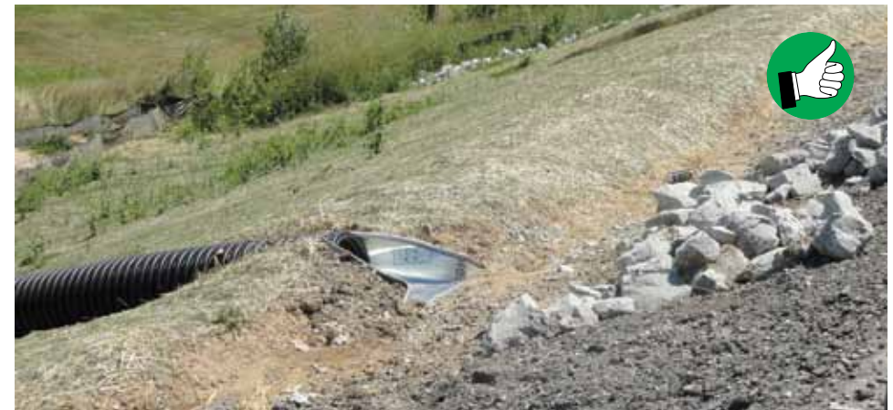
Good example of slope drain diversion channel and inlet.
