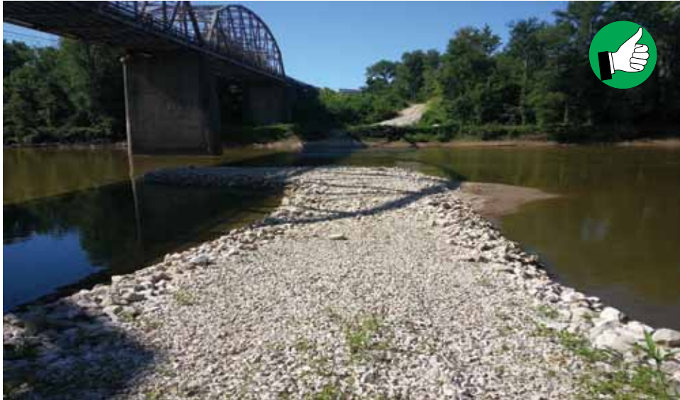
Permitted aggregate cofferdams used as working platforms.
