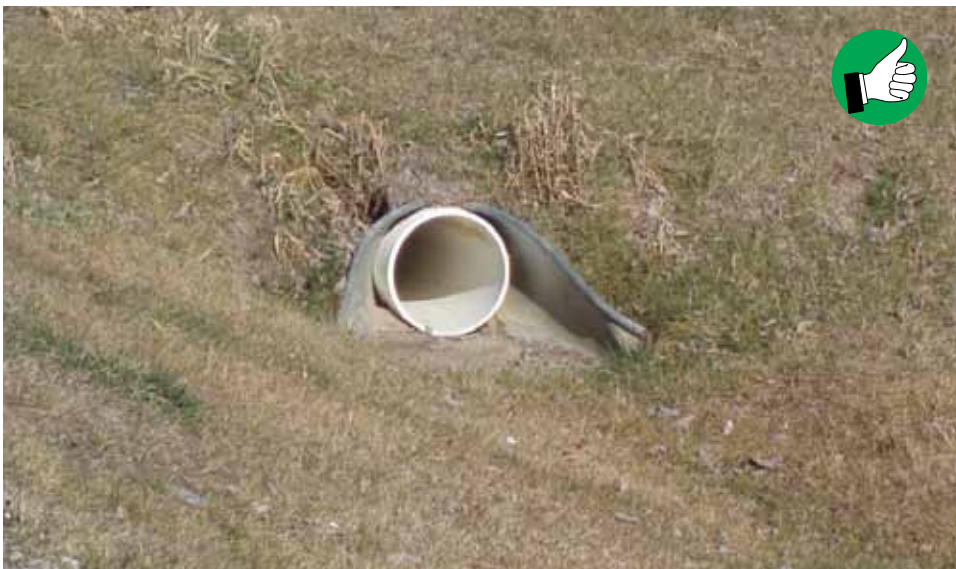
Pipe does not need riprap for permanent inlet protection because permanent vegetation was established for stabilization and velocity is low.
