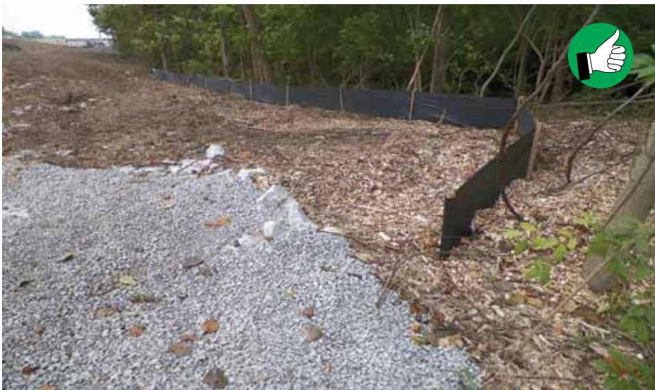
“J” hook the end of the silt fence uphill to prevent water from bypassing fence.
