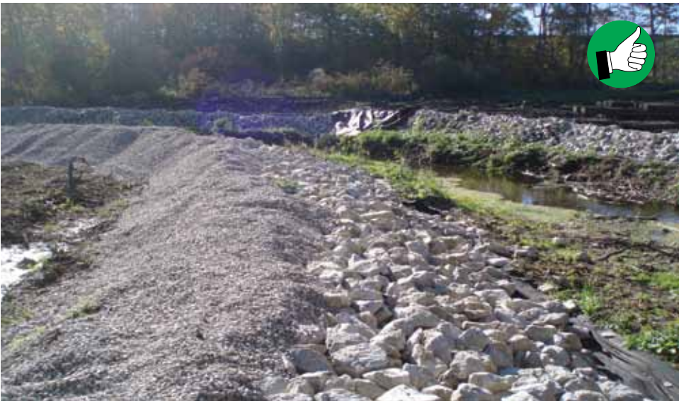
Filter berm protecting creek with geotextile, revetment riprap and filter stone. Note existing vegetation left in place between filter berm and waterway.
