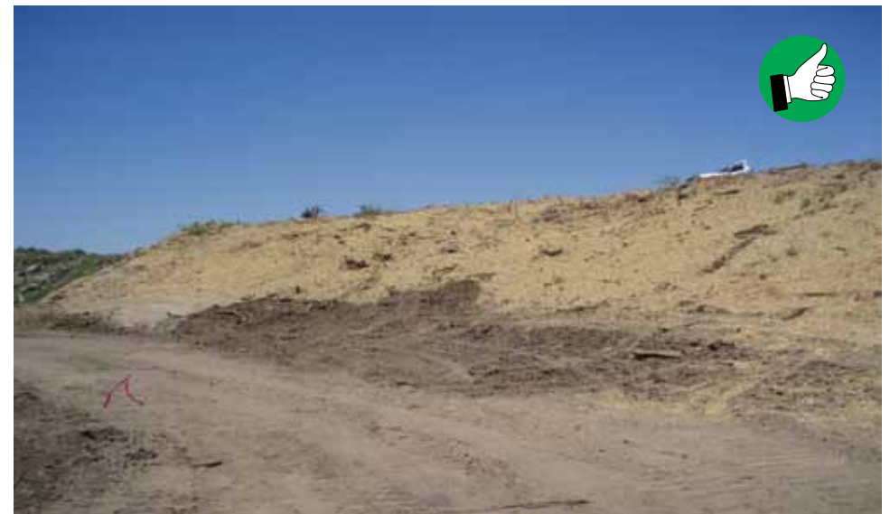
Stockpiled soil protected with mulch.
