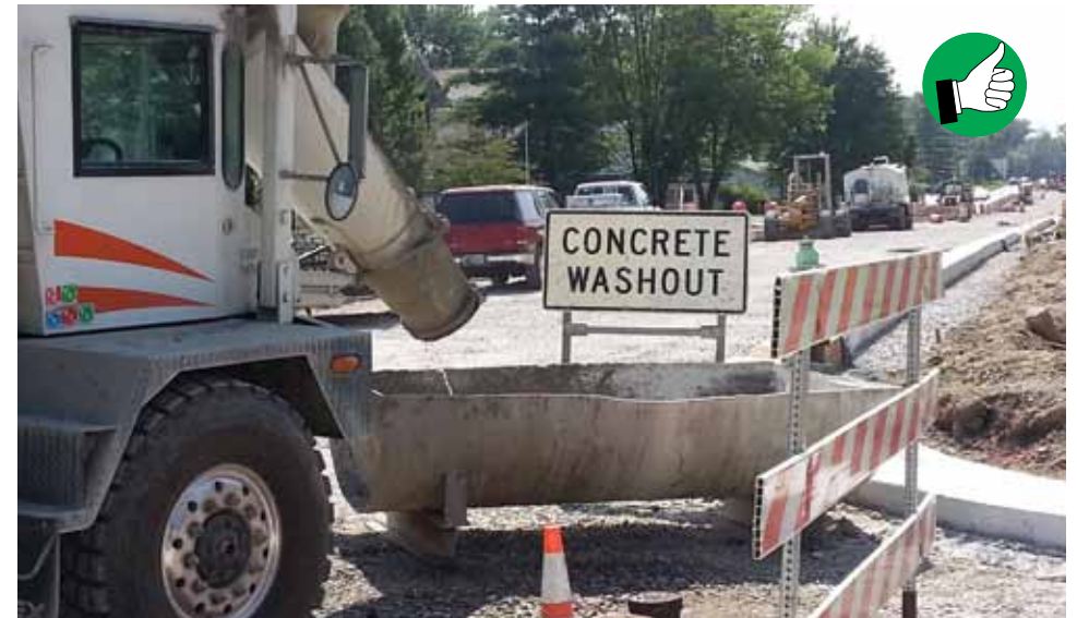
Concrete washout contained within a container with signage.
