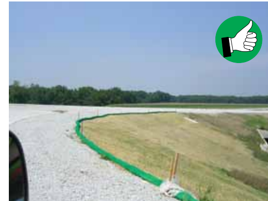
Filter socks can be used on the edge of pavement to slow water before vegetation is established.
