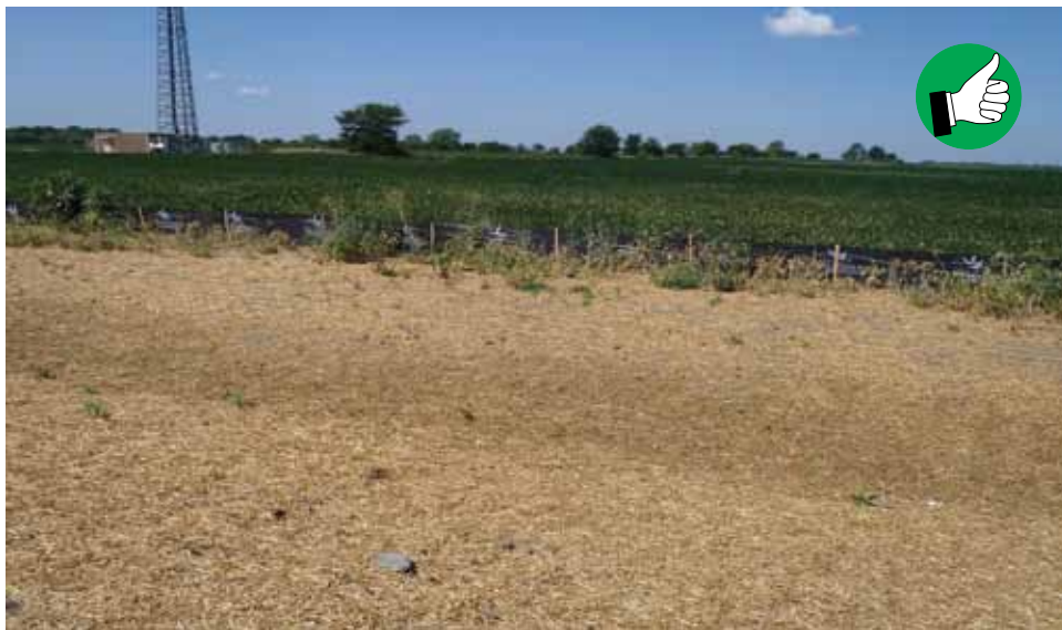
Mulch applied adequately and uniformly.
