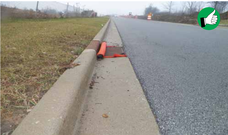
Inlet bag protection can be used on curb inlets with active traffic. Maintain bags after each storm event. Bags can get heavy and hard to maintain when very full.
