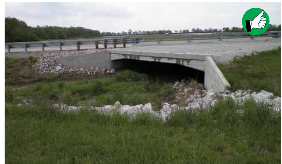
Permanent inlet protection includes wing walls and riprap protection.
