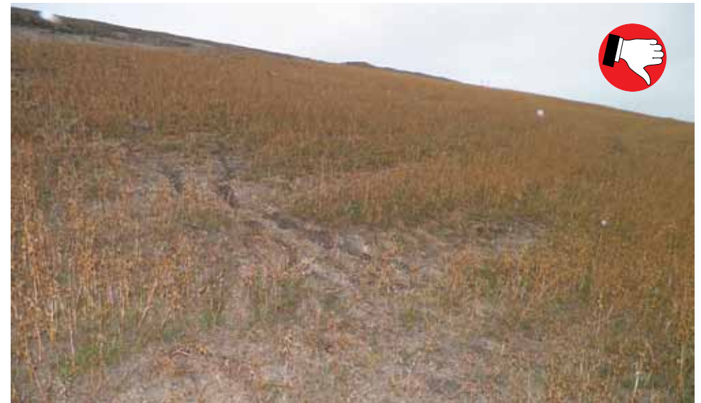
Temporary seeding on long steep slope requires maintenance.
