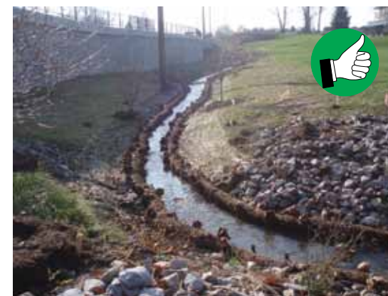
Filter socks used for channel stabilization.
