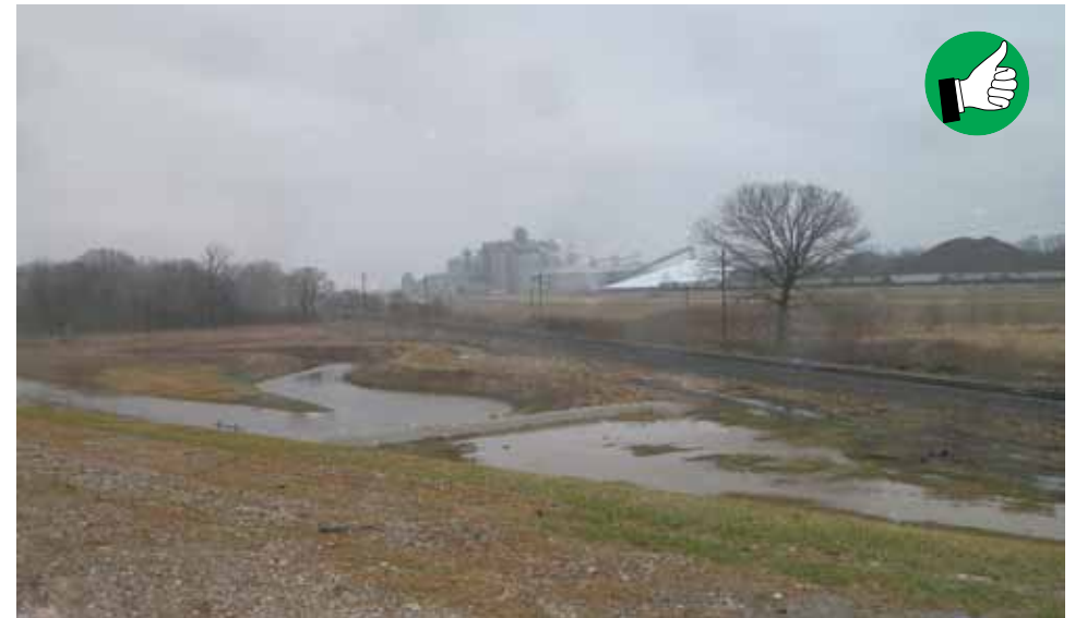
Filter berm protecting newly constructed stream mitigation.
