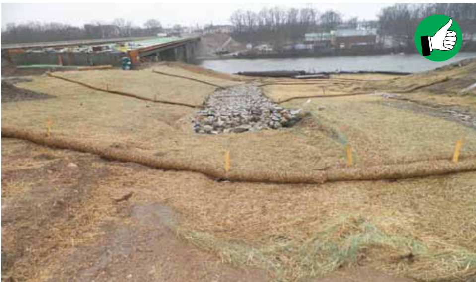
Filter socks can be placed horizontally across a slope to shorten a slope's length and prevent rill and gully erosion.
