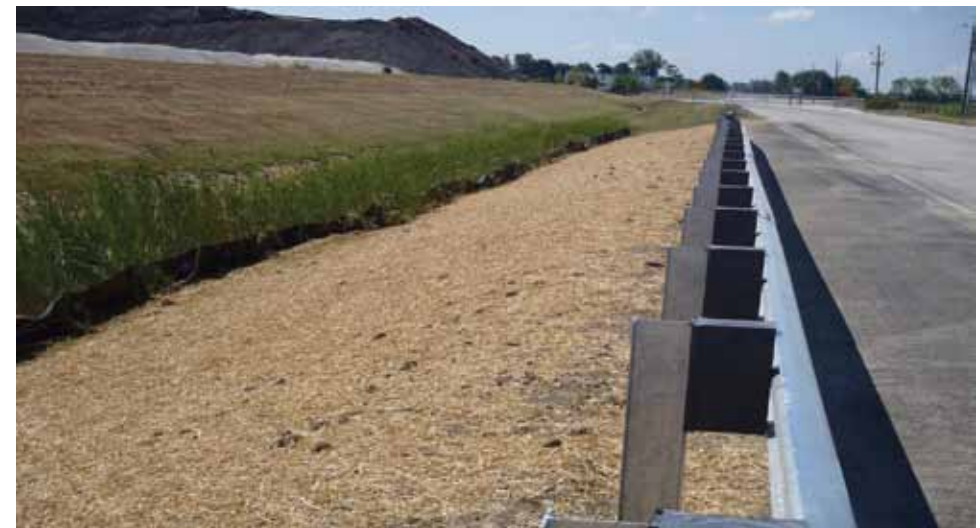
Silt fence and mulch protecting a wetland (hot spot).
