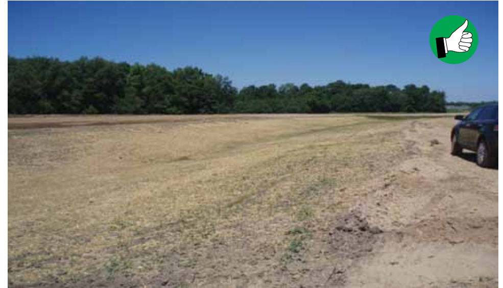
Early stages of temporary vegetation providing slope stability.
