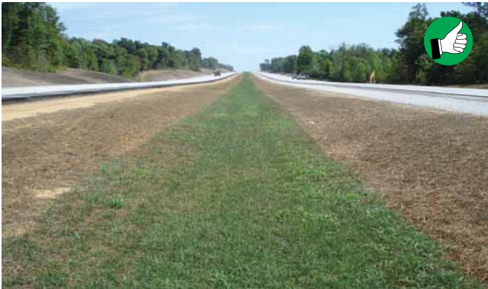
Permanent sod installed in concentrated flow area in median.
