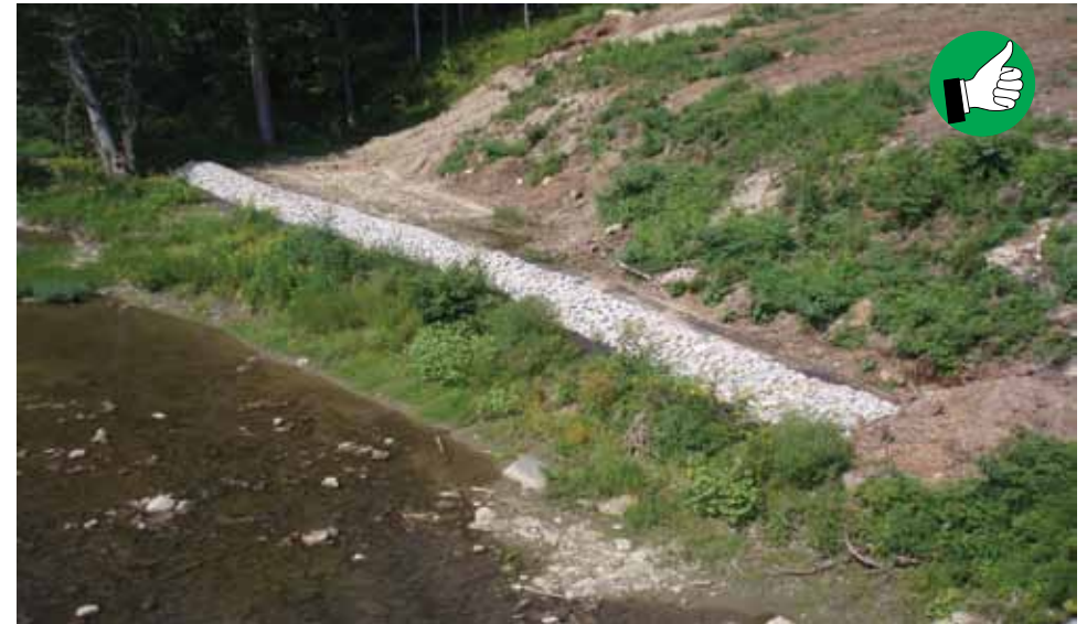
Filter berm protecting creek from long fill slope. Note existing vegetation left in place along creek bank.
