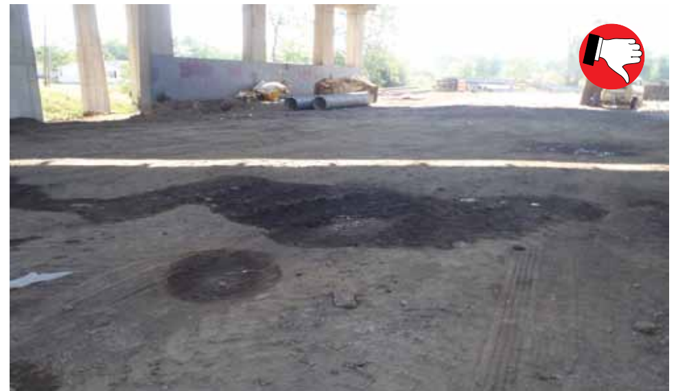
Prevent fuel or other toxic spills. Locate spill cleanup kits in accessible areas and clean up immediately.
