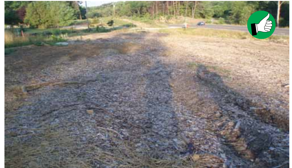
Wood chips from tree clearing used as erosion control.
