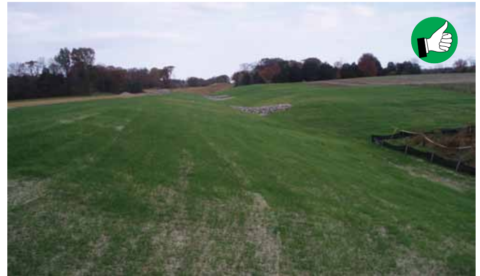
Temporary seed or permanent seed as early as possible to reduce dust on a construction site.
