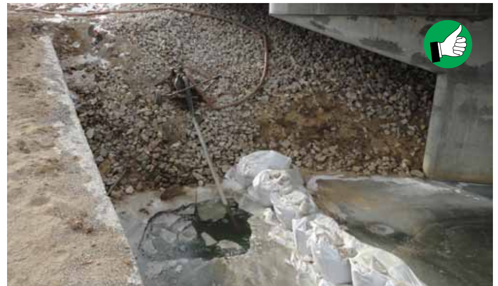
Sand bags can be used as cofferdams.
