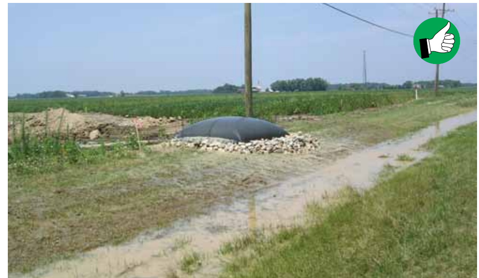
Filter bag placed on flat surface away from sensitive environments.
