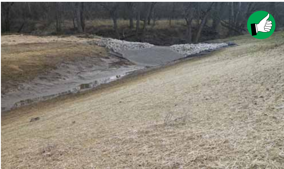
Sediment trap placed at the end of the ditch right before a waterway.
