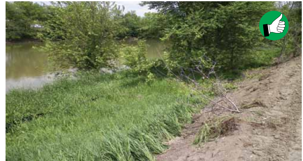
Good example of vegetative filter strip (and silt fence) protecting the waterway from sediment.
