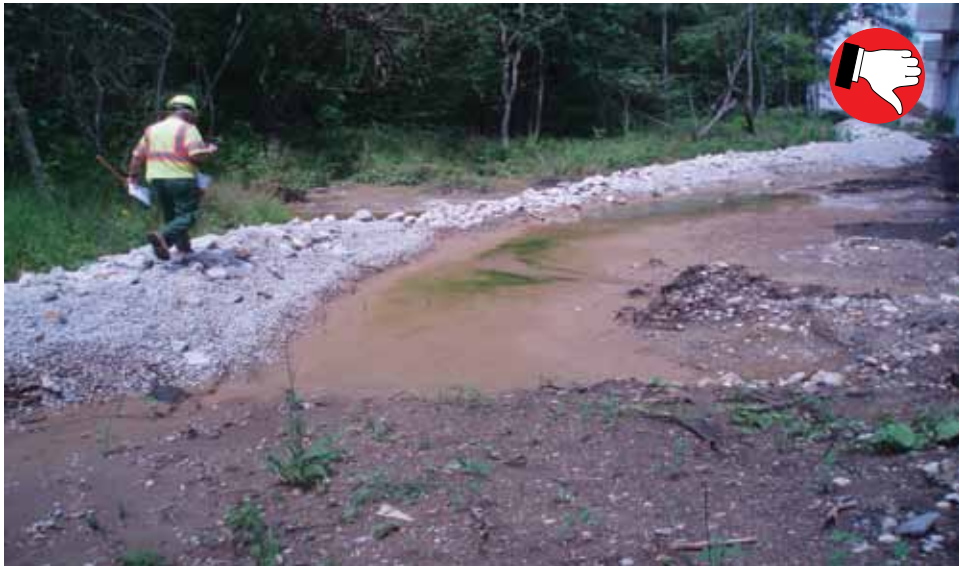
Filter berm after a large rain event that needs maintenance.
