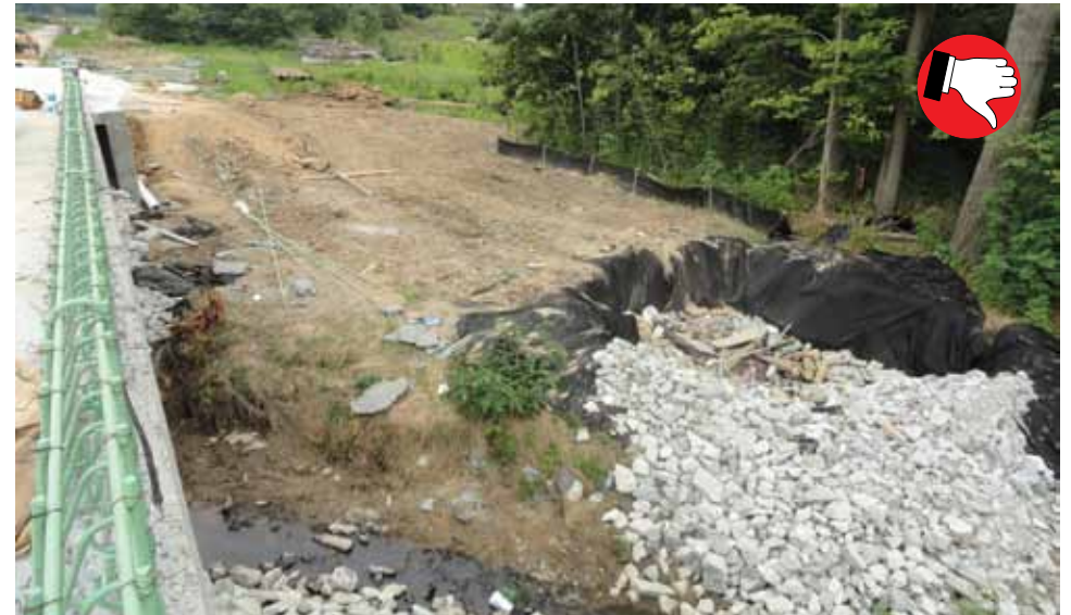
Keep construction debris contained in designated areas, away from hot spots and BMPs.
