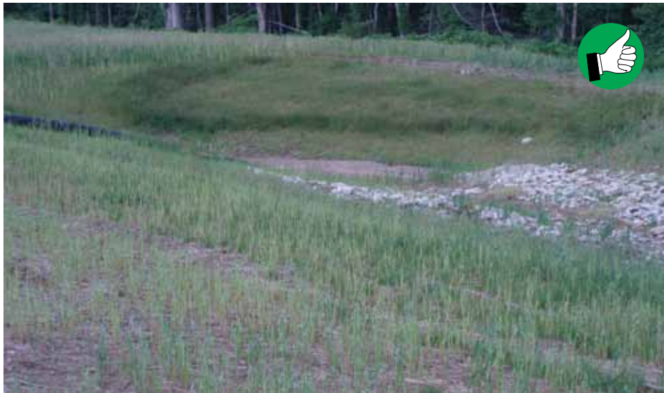
Temporary vegetation and slope drains providing slope stability.
