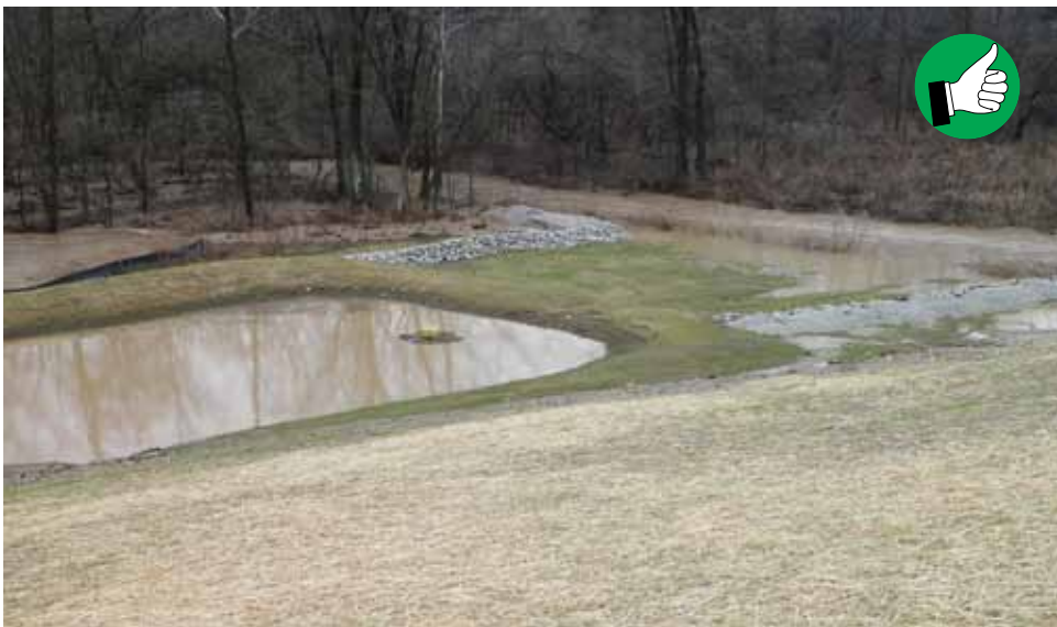
Sediment basin stabilized with vegetated banks, riser pipe and stable overflow.
