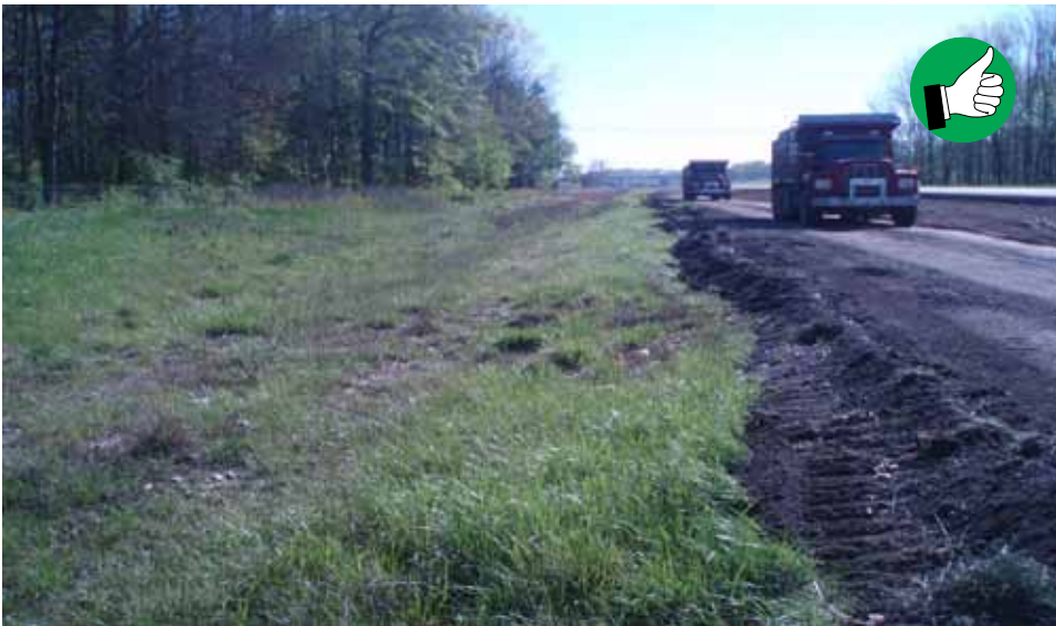
Existing vegetative buffer along and within the ditch.
