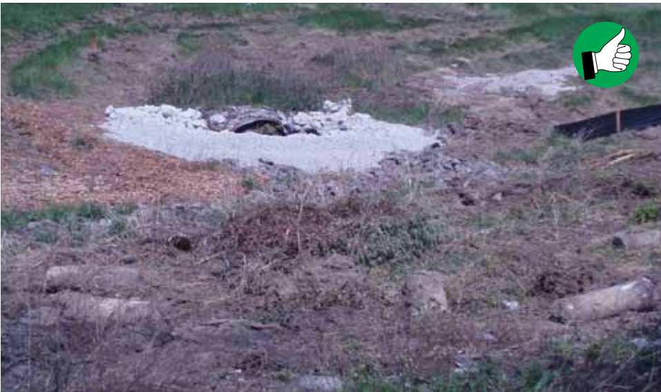
Inlet protected from sediment with filter stone surrounding riprap.
