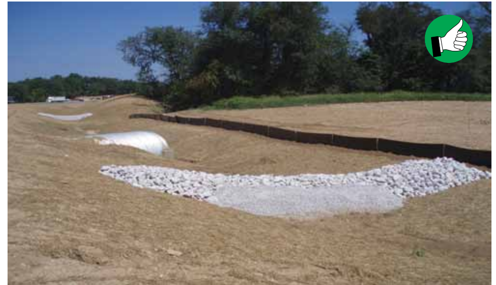
Check dam shaped correctly with low weir in the middle and tied into the slopes.
