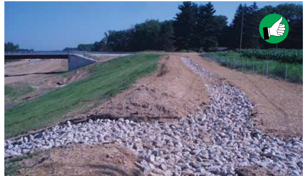
Example of permanent Diversion Interceptor installation
