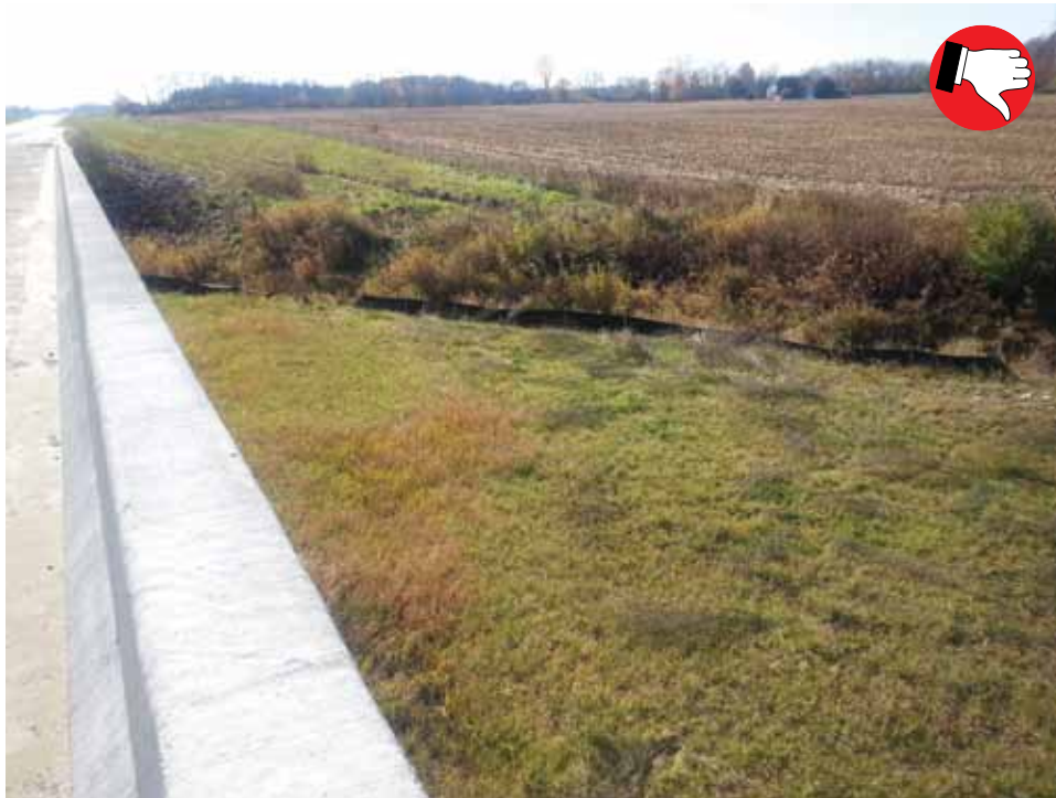
All temporary erosion and sediment control measures must be removed prior to issuing the NOT. Although the site is stable and more than 70 percent uniform density of vegetation, silt fence was left along the creek.
