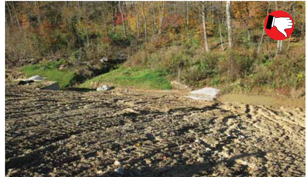
Trap placed too far away from waterway, should have a stable outlet to the creek and needs maintenance.
