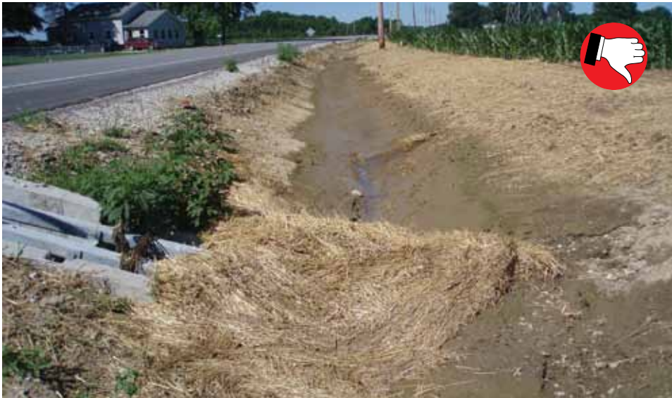
Mulch is not an appropriate protection for seed in concentrated flow areas.
