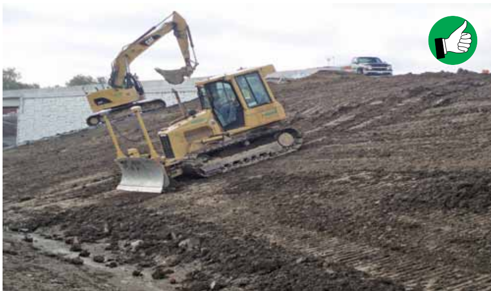
Operate bulldozer or other tracked vehicle up and down slopes before seeding to create tread-track depressions for catching and holding seed.
