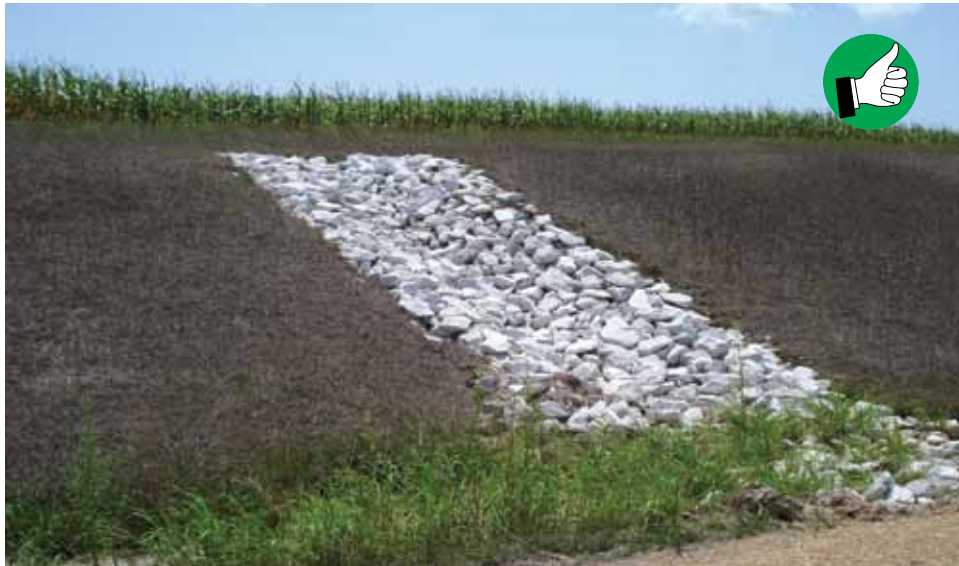
Good example of placement of a rock chute to help with runoff from an adjacent farm field.
